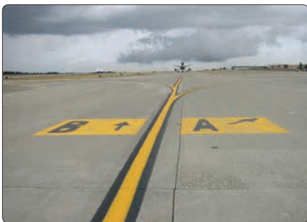
Figure 14-19. Surface painted taxiway direction signs.
