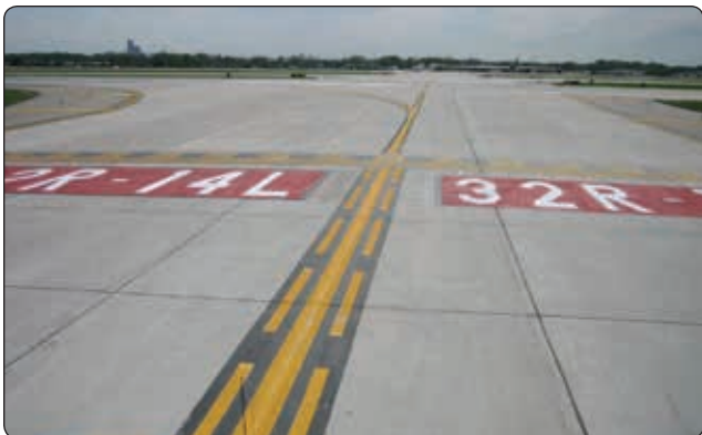
Figure 14-12. Surface painted runway holding position signs for Runway 32R-14L along with the enhanced taxiway centerline marking.
