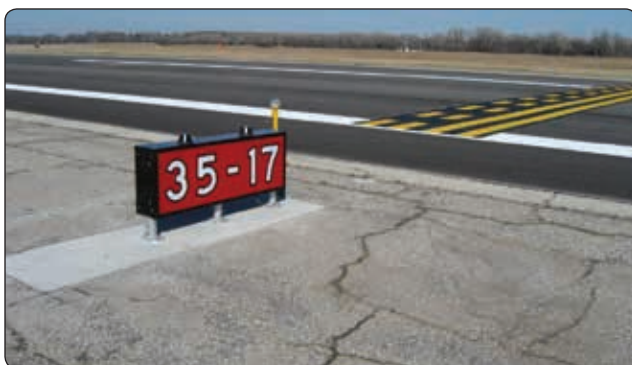
Figure 14-17. Runway holding position sign and marking for LAHSO.
